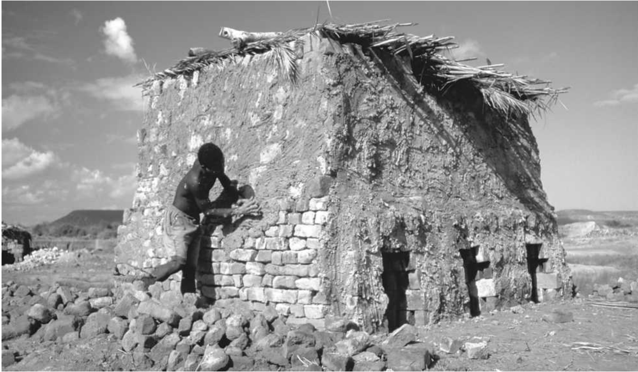
In rural areas people must rely on local materials when building homes and walls. This oven is constructed of mud bricks and a plaster made of hard drying mud.
